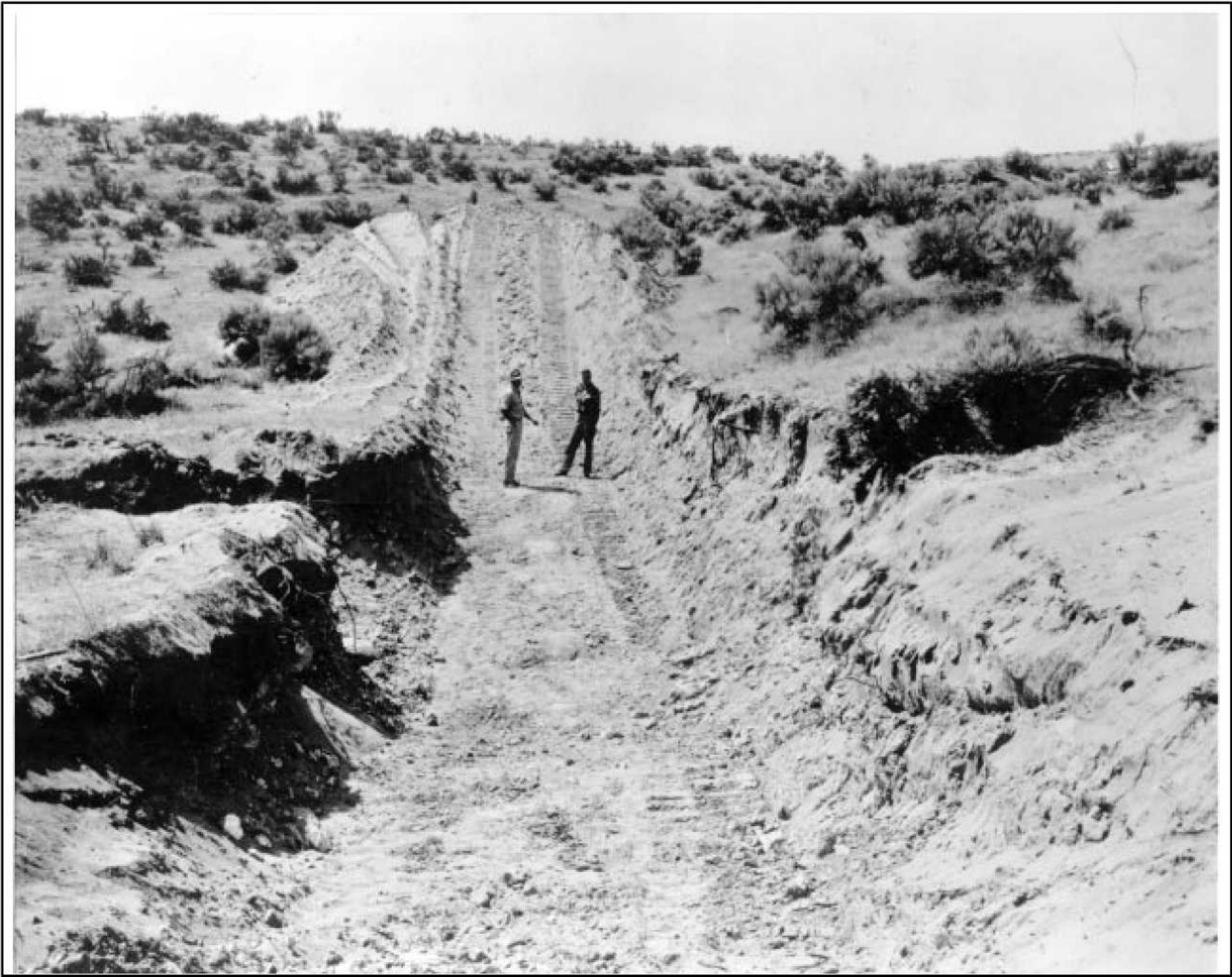
Figure 2-19.—Shallow test trench excavated by bulldozer.
